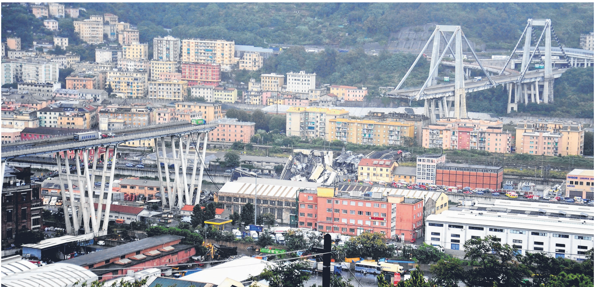
A 50m-high section of Genoa's Morandi Bridge crashed down in the rain onto the roof of a factory and other buildings, crushing vehicles below and plunging huge slabs of reinforced concrete into the riverbed. PHOTO: REUTERS
