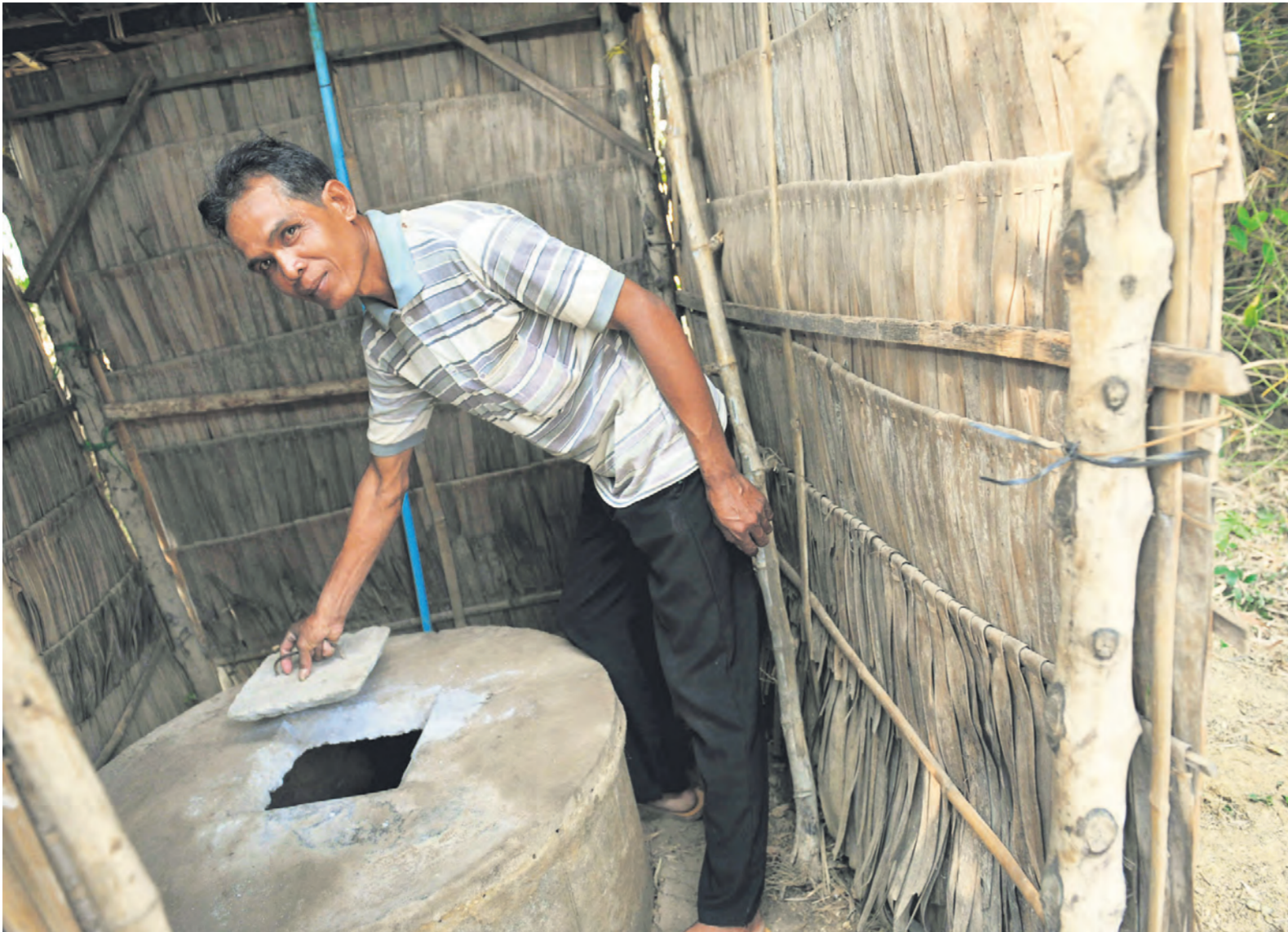
Paddy farmer Nguon Kong showing off his dry pit latrine in the Community Led Total Sanitation village of Kampong Speu. The latrine, which is essentially a hole in the ground reinforced with a concrete ring, does not give off a foul odour. Users add ash after each use to keep the smell at bay.
