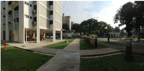
TOP Proposed site HDB void deck at Chong Boon, Ang Mo Kio
